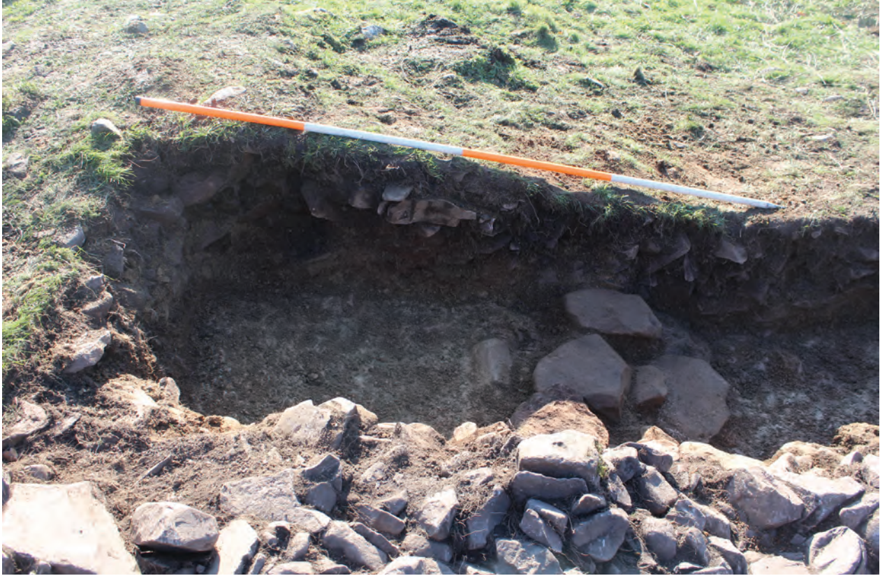
Figure 34 Stone revetment kerb (2016), facing south-west. Scale 2 m
